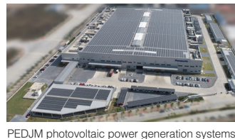
PEDJM photovoltaic power generation systems
