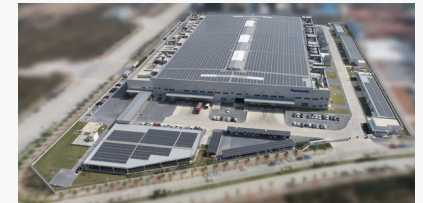
Photovoltaic power generation systems at PEDJM
