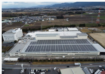
Photovoltaic power generation system at Youkaichi site, LVBD, Panasonic Living Appliances and Solutions Company
