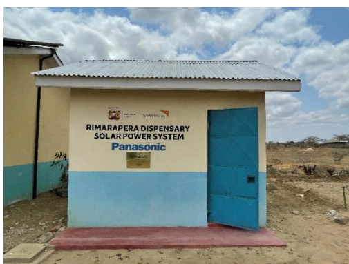
The PSS building
