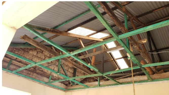
Former roof under renovation
