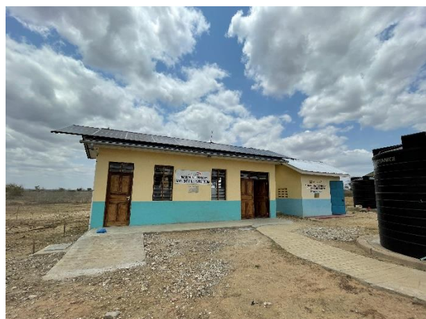
Solar panels installed on the roof of delivery room
