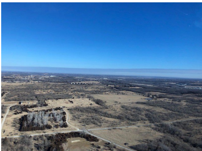
Construction site of new manufacturing facility in Kansas
