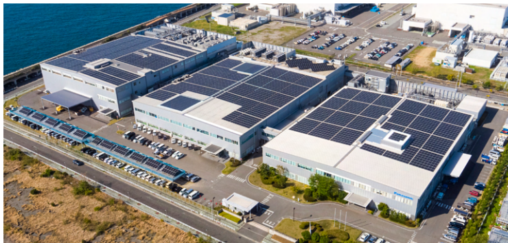
Photovoltaic power generation system at the dry batteries factory in Nishikinohama
