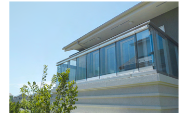
"Energy-generating glass" in harmony with the town and everyday life installed at a model house at Fujisawa SST for demonstration test
