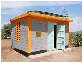
A photovoltaic and energy storage system was installed at the primary school and health clinic.
