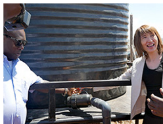
The solar-powered water pump started running.
