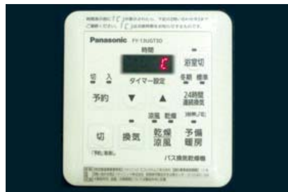
A "C" flashes on and off in the remote control display when an inspection is due
