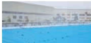
Recycled wastewater is sprinkled on the roof of the plant to lower the surface temperature of the building.
