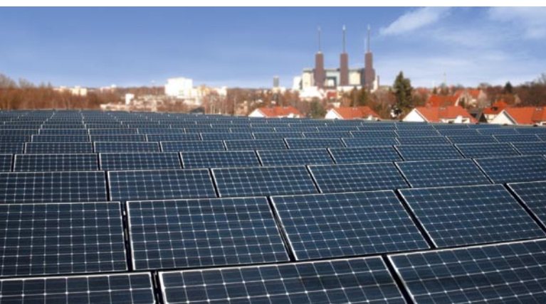
HIT solar-cell modules installed on the roof of the City Gymnasium in Berlin, Germany.
