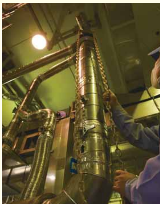
Opening/closing the upper valve using a chain, thereby reducing the use of dry air
