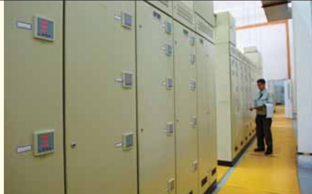
Visualizing total power consumption at the factory using 270 power meters managed in the power distribution room
