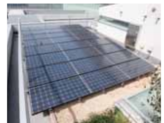
Solar power generation system (Output: 5,040W)
