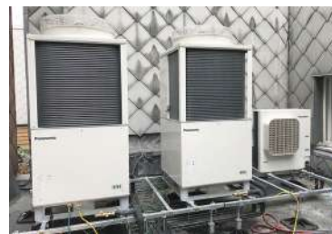
Example of two 10-horsepower freezer and one two-horsepower freezer at Carrefour Express (small stores)
