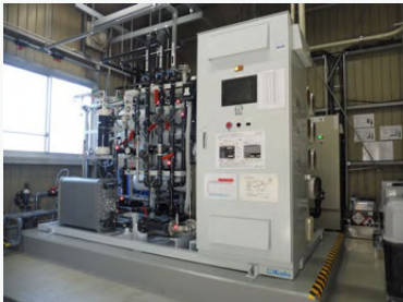
Water purification system with electrical resin regenerator
