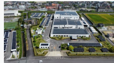
Photovoltaic power generation systems at Saga Site, Panasonic Industry
