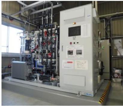
Water purification system with electrical resin regenerator
