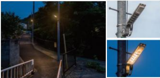
Street lights in Zushi City are replaced with firefly-friendly LED lights
